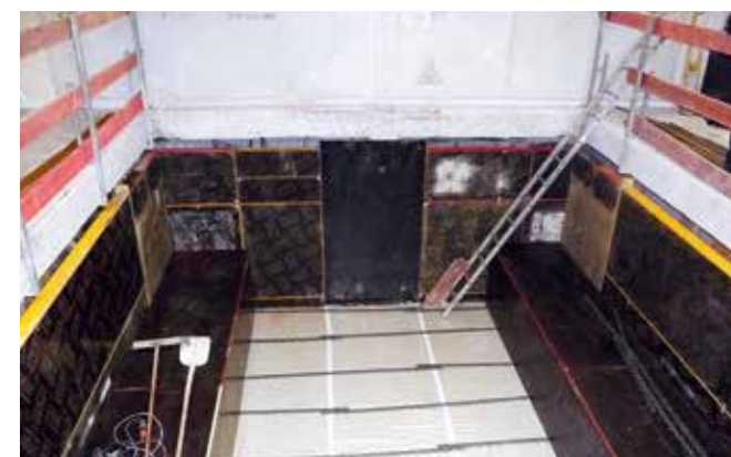
Formwork on the support foundation
