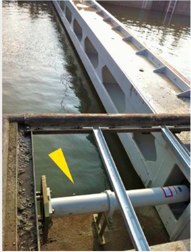
Heavy safety shock absorbers, which are specially designed for this application, are able to brake in lock masses of up to four million kg
